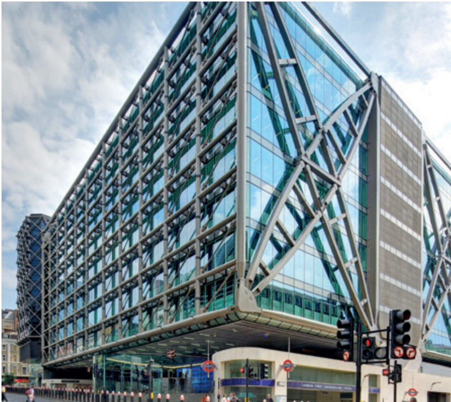
ASD0540-S tie bars M76 to M160 were used as the tension elements in the trusses to form part of this unique and structurally demanding London office building at Cannon Place.
